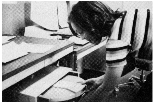
Figure 26.4. Inserting the disk pack in the Dynabook.
